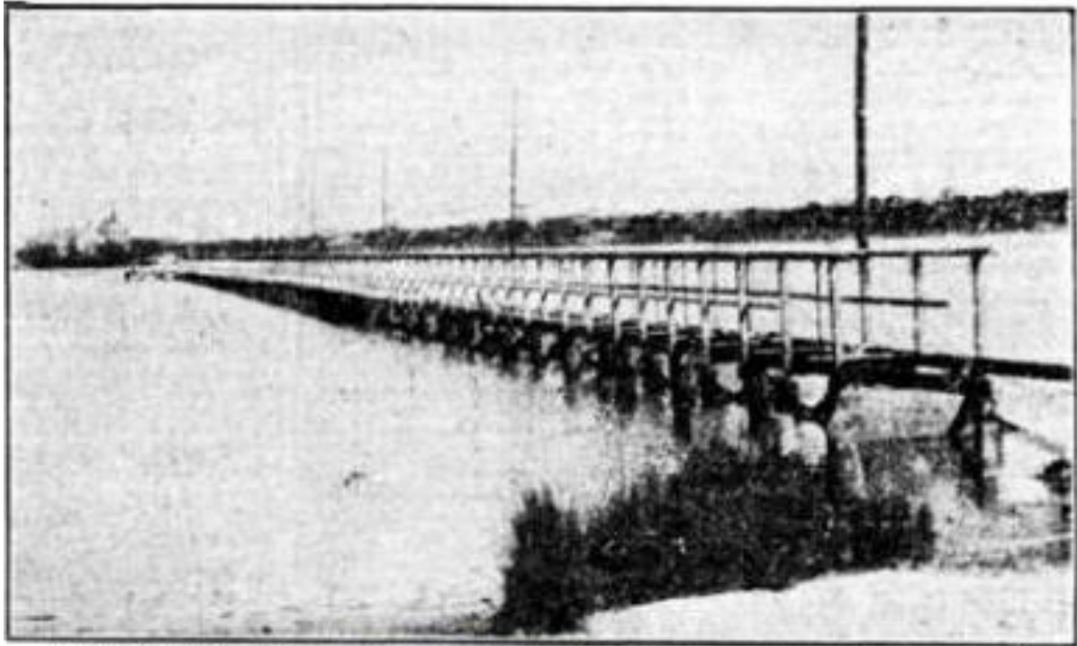
A GENERAL VIEW OF THE MAYLANDS JETTY , which has been rendered unfit for use. The planking at the shore end has been entirely removed, and it would be necessary to wade through mud to reach even the skeleton of the main structure.—“The Daily News” special photograph.
