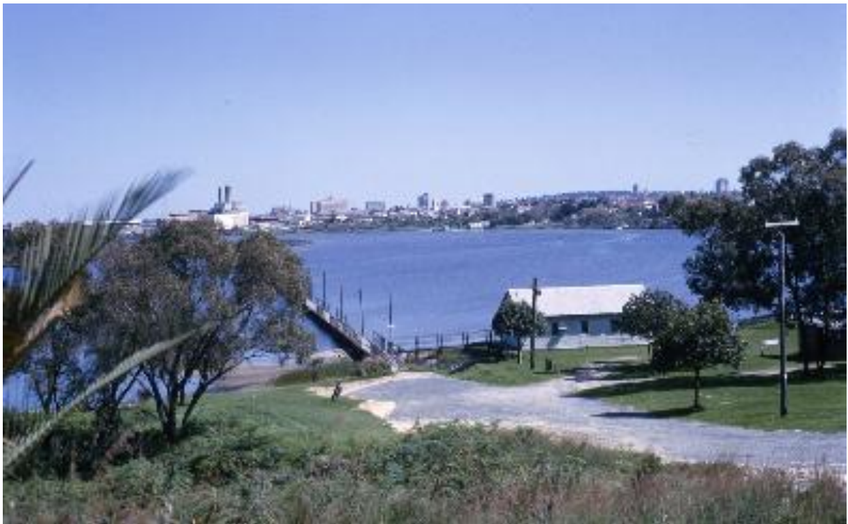
A GENERAL VIEW OF THE MAYLANDS JETTY , which has been rendered unfit for use. The planking at the shore end has been entirely removed, and it would be necessary to wade through mud to reach even the skeleton of the main structure.—“The Daily News” special photograph.
